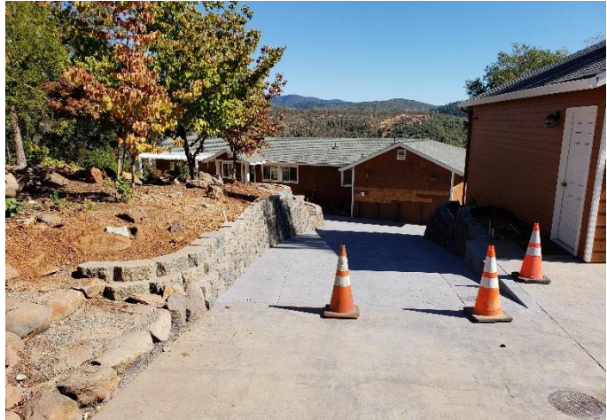
(Retaining walls and corrected driveway grade)
