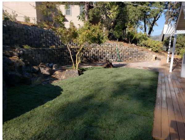
Oct. 25 — Newly installed sod covering the irrigation system
